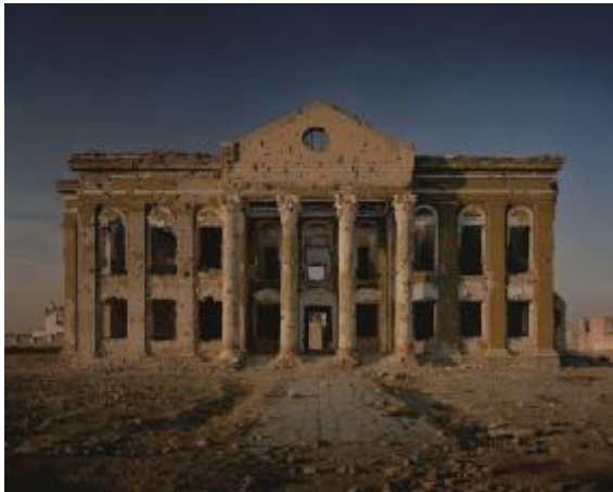
Bild 2 Simon Norfolk A government building, close to the former presidential palace at Darulaman, destroyed in fighting between Rabbani and the Hazaras, 2001 © Simon Norfolk
